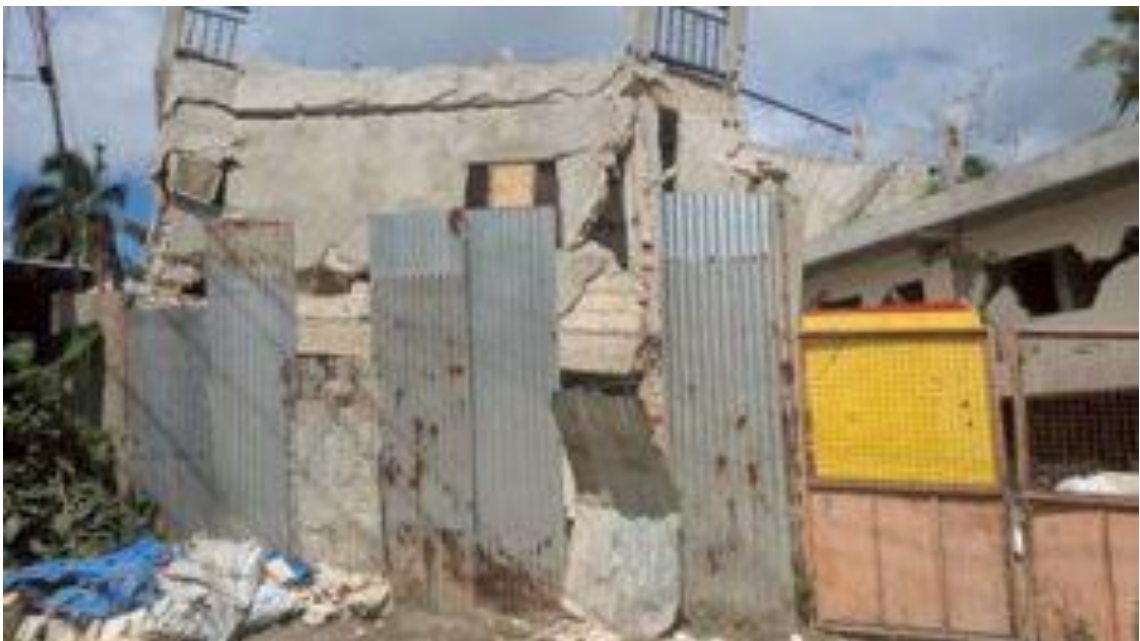
Photo 2: Damage to private properties in the town center.
